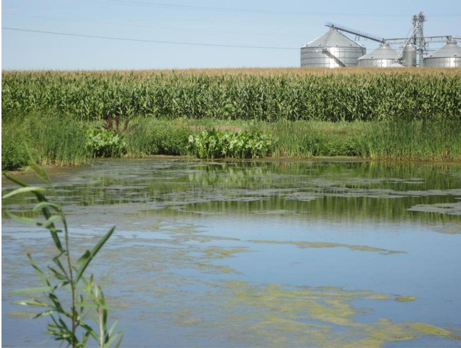
The stormwater treatment pond/Wetland A looking north. This pond was constructed in an upland area after 2010. It has taken on wetland characteristics but was clearly built for the purpose of treating stormwater from the surrounding development.
