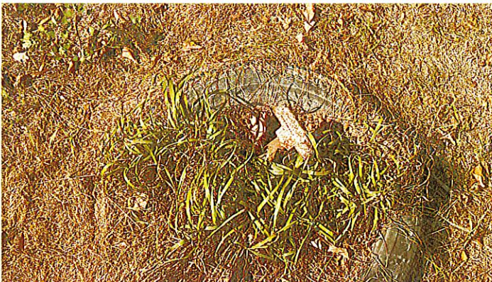
12. Photograph shows the apparent vent pipe observed to the south of the farmhouse.
