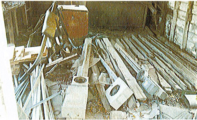
14. Photograph shows electrical material present in one of the farmstead buildings.
