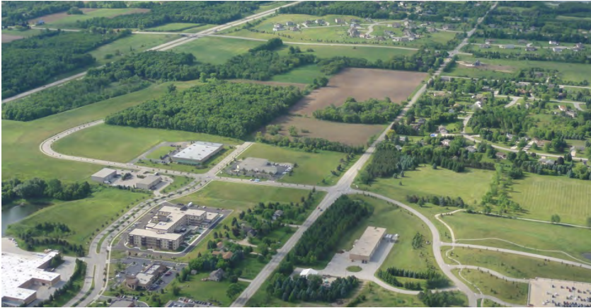
West Bend Corporate Center Southeast view
