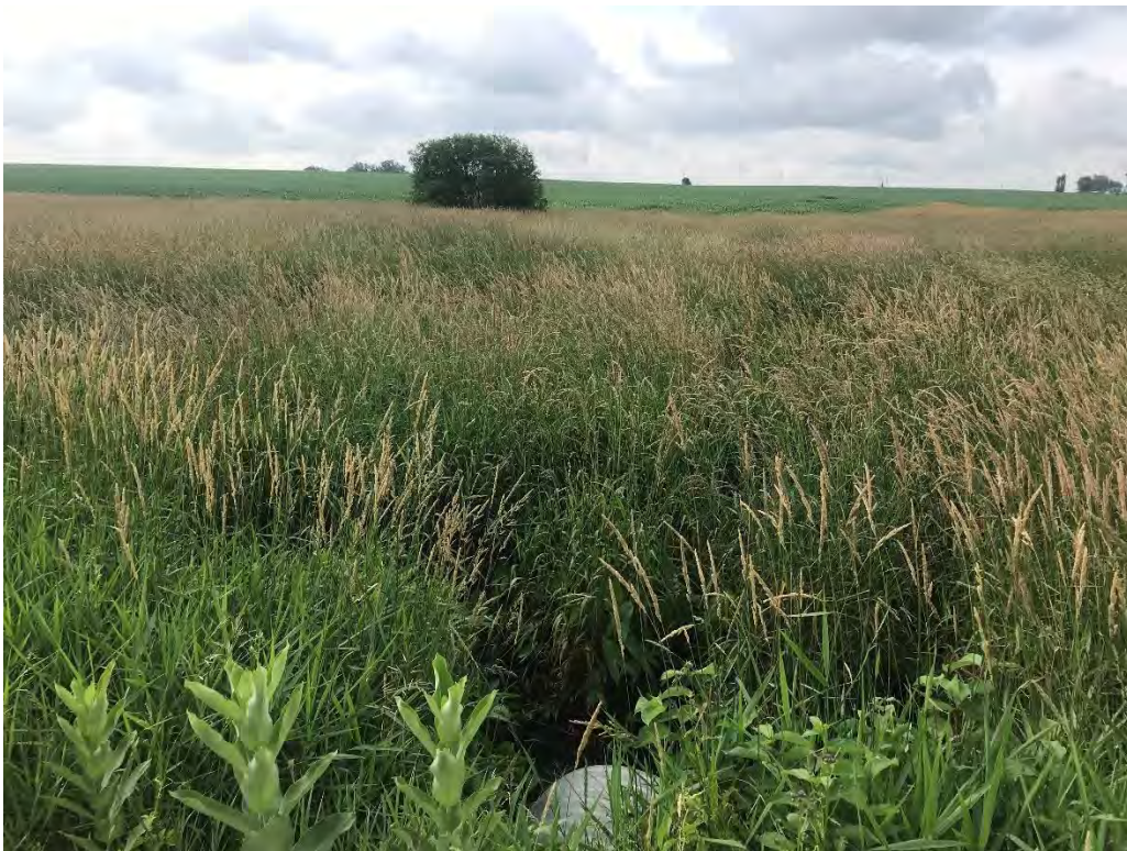
Photo 14: Looking south from 80 th Street at Area A. Culvert with standing water flowing north.
